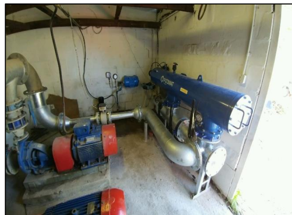
The new filter in the pump house
