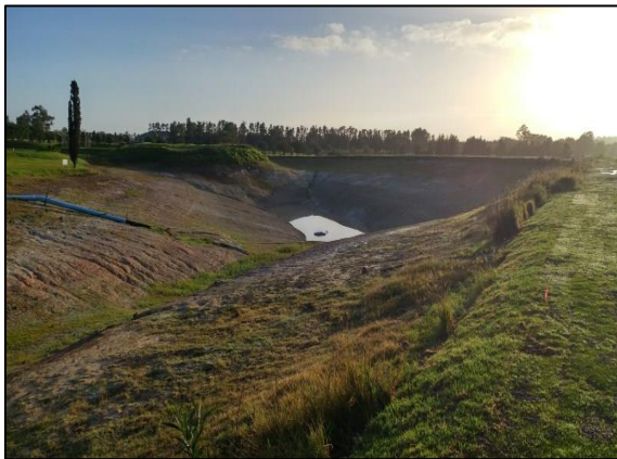
14 th dam in June
